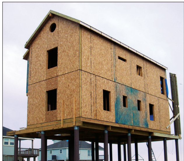
Figure 2. Construction of a Structural Insulated Panel house.
