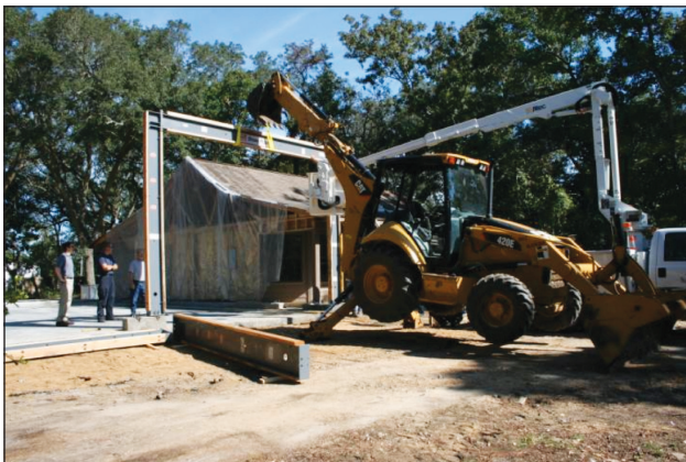
Figure 4. Installation of a prefabricated ordinary moment frame.
