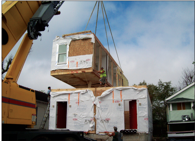
Figure 1. Construction of a modular home.
