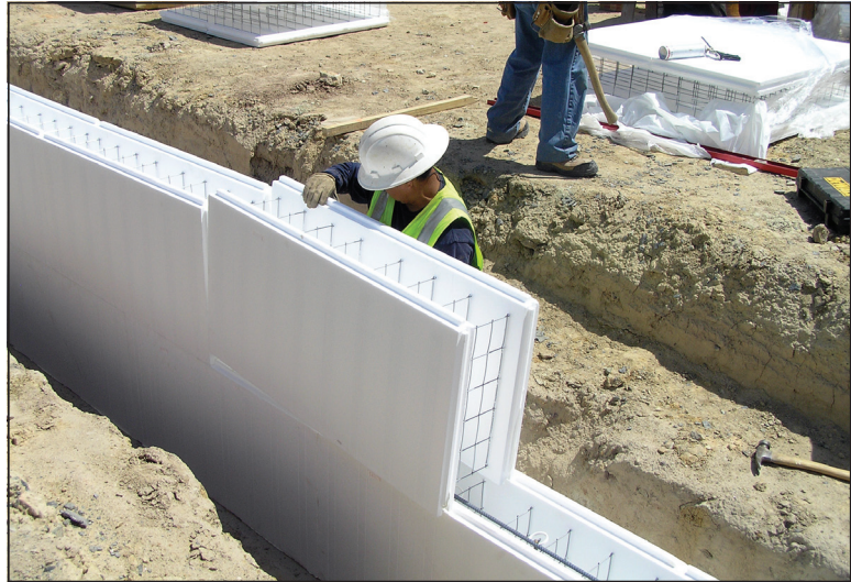
Figure 3. An example of ICF walls and reinforcing steel prior to placement of the concrete. The forms are left in place following placement of the concrete.
