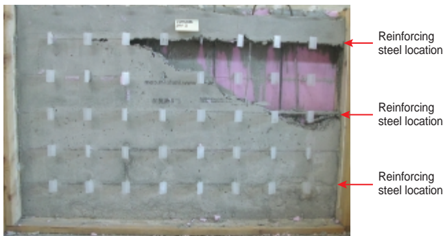
Figure 17. Flat-panel ICF with medium-low slump concrete vibrated with a reciprocating saw. (IMG13349)
