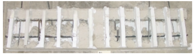
Figure 22. Flat-panel ICF lintel with low slump concrete and no mechanical vibration. (IMG13354)
