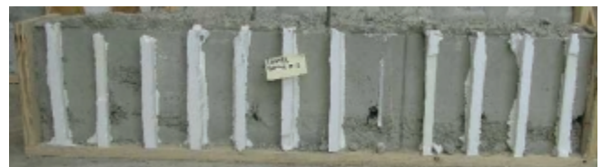
Figure 27. Flat-panel ICF lintel with medium-high slump concrete (no mechanical vibration). (IMG13375)
