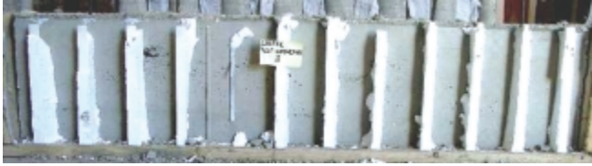
Figure 28. Flat-panel ICF lintel with high slump concrete (no mechanical vibration). (IMG13377)
