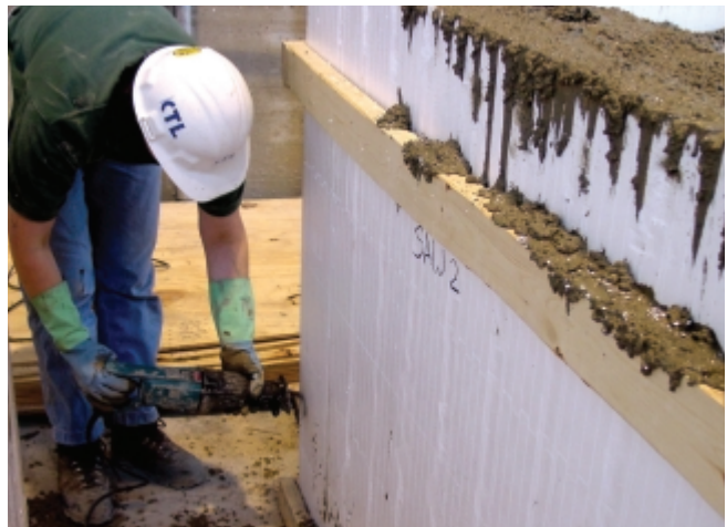
Figure 8. Concrete consolidation using a reciprocating saw with a bent blade. (IMG13340)
