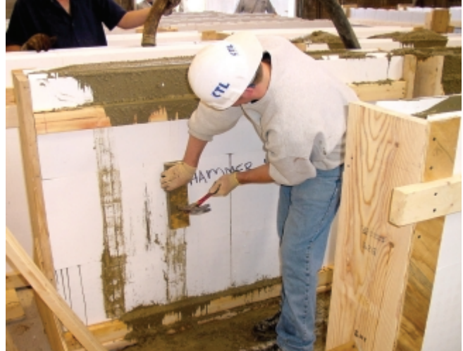
Figure 7. Concrete consolidation using a hammer and block of wood. (IMG13339)
