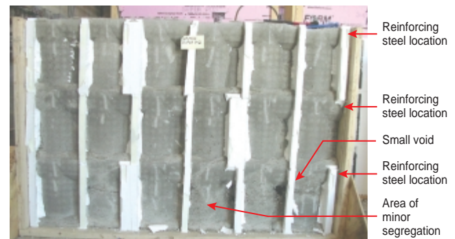
Figure 14. Waffle-grid ICF with medium-high slump concrete and no mechanical vibration. (IMG13346)
