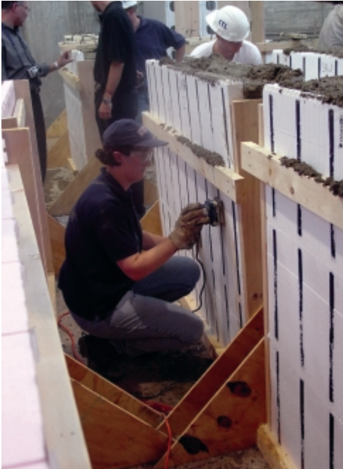
Figure 9. Concrete consolidation using an orbital sander. (IMG13341)
