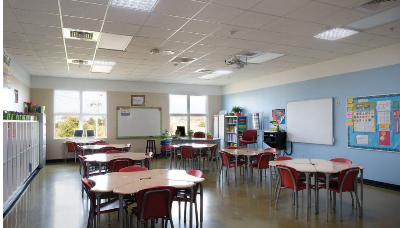
The north-facing classrooms don't have lightshelves. In addition to the view glass, four supplemental tubular daylighting devices provide a source of natural light.
