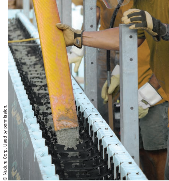
Richardsville was constructed using insulated concrete form (ICF) walls that enhance the building's thermal envelope.
