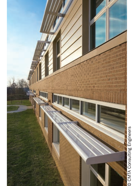
The south side of the building has exterior lights/shelves to direct sunlight further into the classroom.
